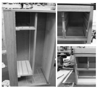
Use clamps to clamp the chest together while the glue dries. Check the cabinet for square before glue cures. Adjust if required.
